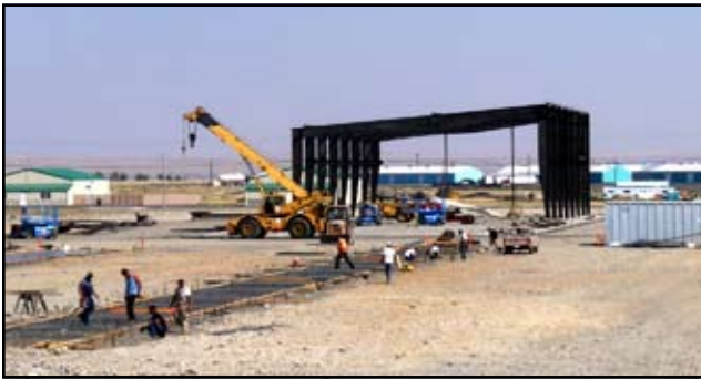
Construction on the Katana facility in Ephrata
