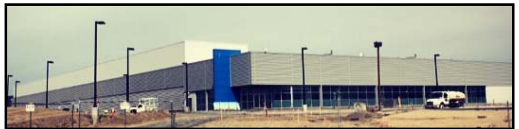
Vantage Data Center Facility in Quincy
